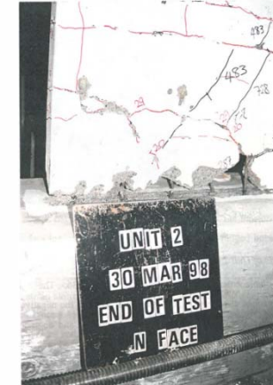
Figure 5.34. Fractured bars at base of Unit 2, end of test.
