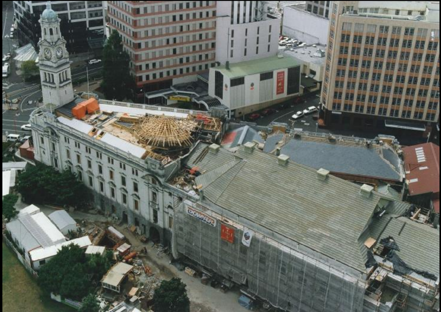
RESTORATION IN PROGRESS 1996
