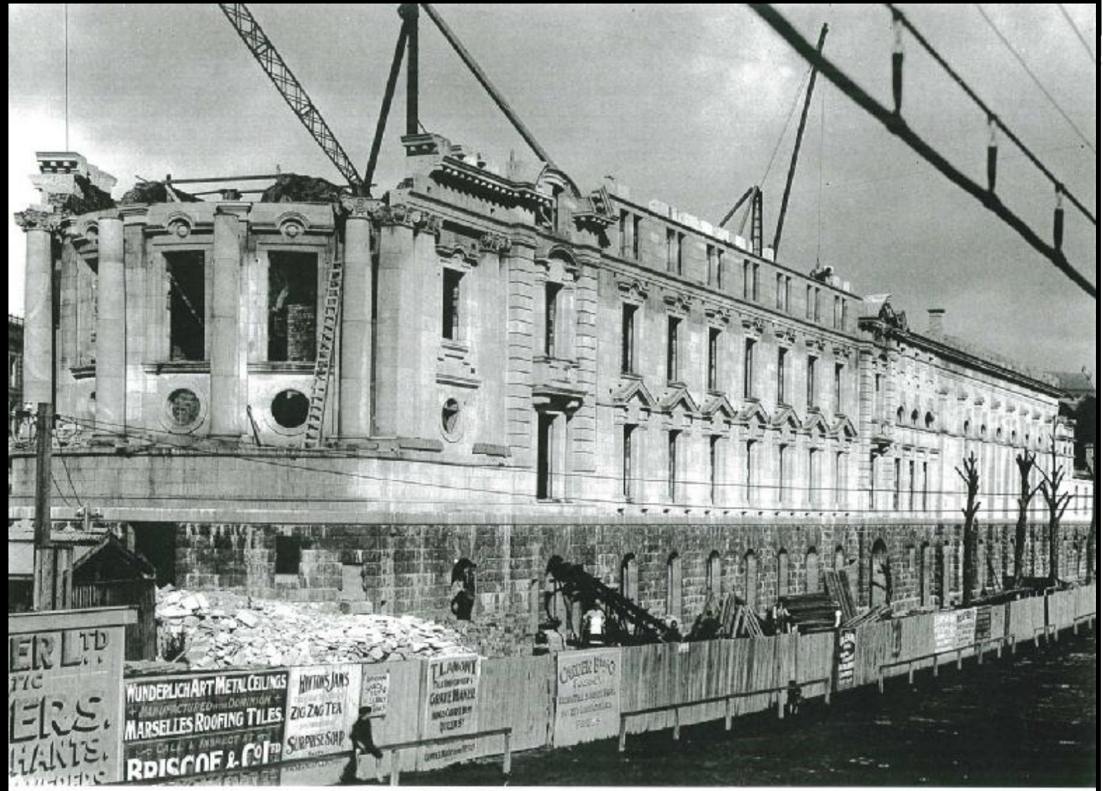
BUILDING IN PROGRESS 1910
