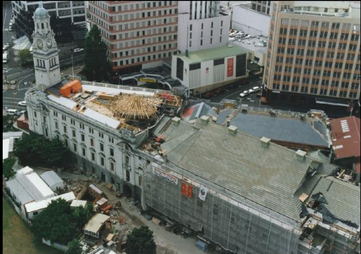
RESTORATION IN PROGRESS 1996
