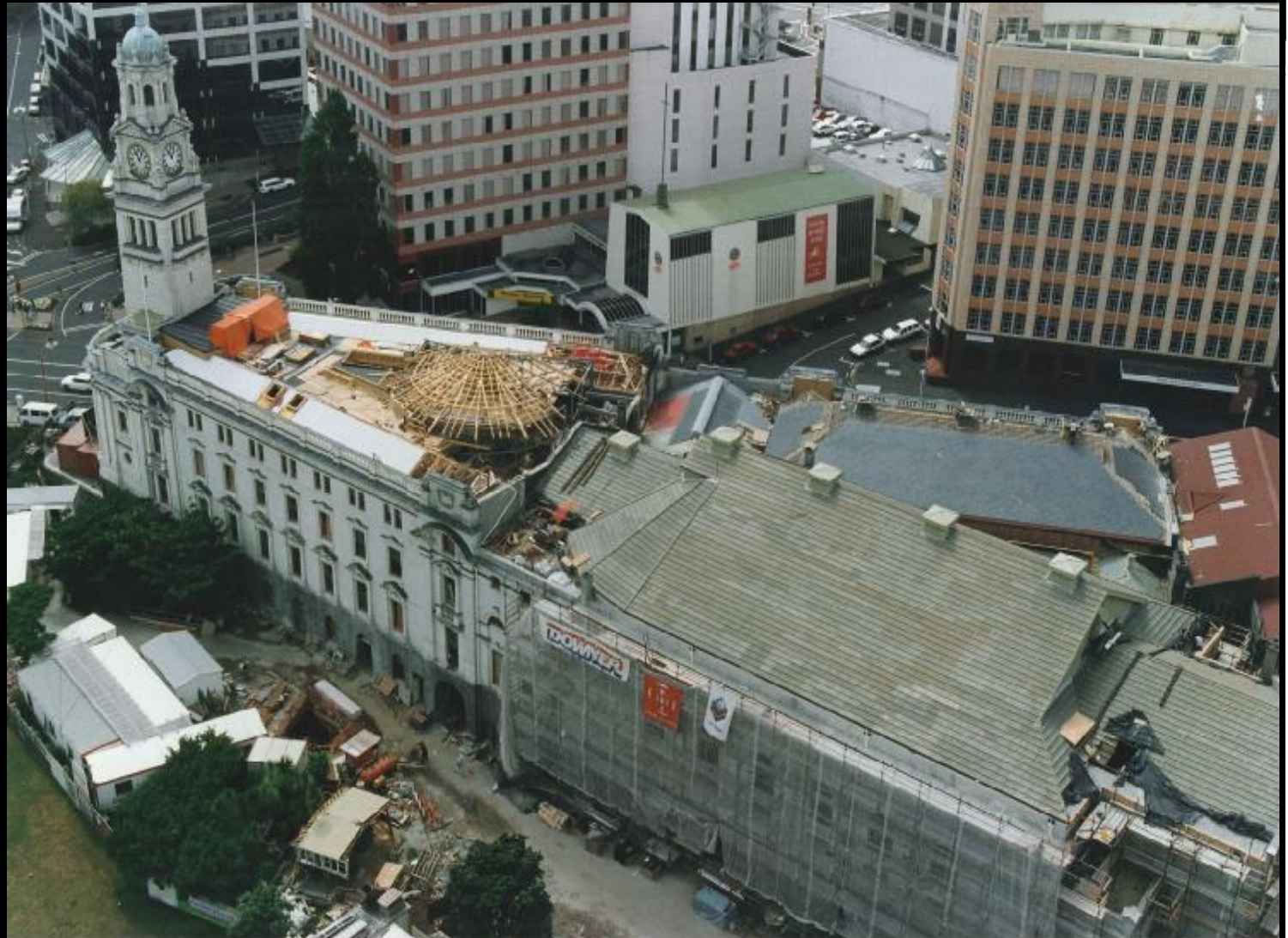
RESTORATION IN PROGRESS 1996
